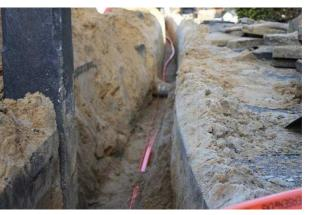
from conduit easily. More importantly is the protection it can provide during future excavation near your facilities. The apparent change in soil condition provides warning that there is a utility buried there. This should not replace the practice of placing warning tape, but rather should serve as a supplement.
