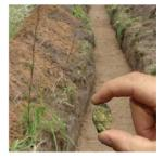
large stones from the bottom of the trench to prevent damage to the conduit. Push some clean fill (fine material, without stones) into the trench to cushion the conduit as it is installed in the trench. Supplemental trenches should be made to all offset enclosure locations. Trench intersections should be excavated to provide adequate space to make sweeping bends in the DuraMultiDB conduit. Fill
